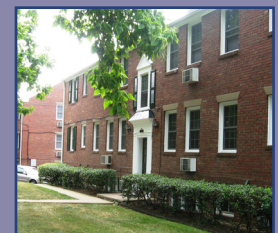
Fairfax Drive Apartments
